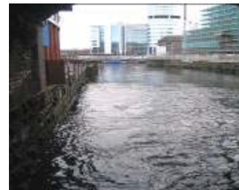
Dark Arches, Granary Wharf
